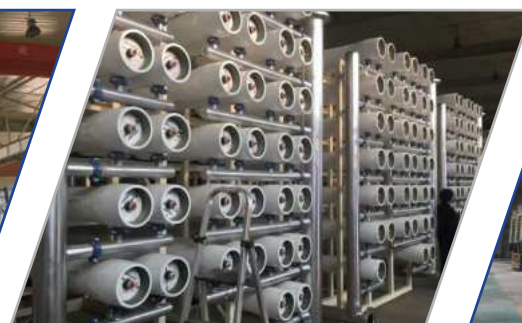
Qingdao wastewater reclamation project. Aug 2016
