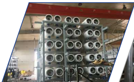
Daya Bay Cnooc's refinery project. July 2016
