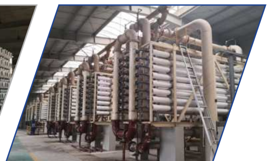
Dalian Hengli petrochemical water treatment project. Nov 2017
